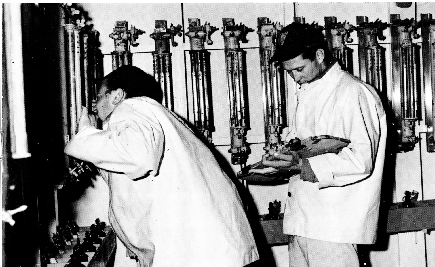
THE TEMPERATURE being read from a precision thermometer attached to a Nansen bottle.
